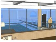
concrete roof slab structures covering the filters, and construction of above-ground building structures over the filters in place of the currently existing underground roof slabs in order to furnish full visibility and access to
